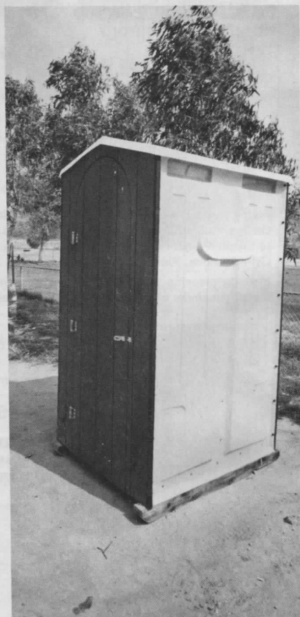
The plastic sides and roof are apparent in this picture of the new unit. Much lighter than the older unit, and easier to transport, the new unit displays some squirrely handling in high, gusting winds.
